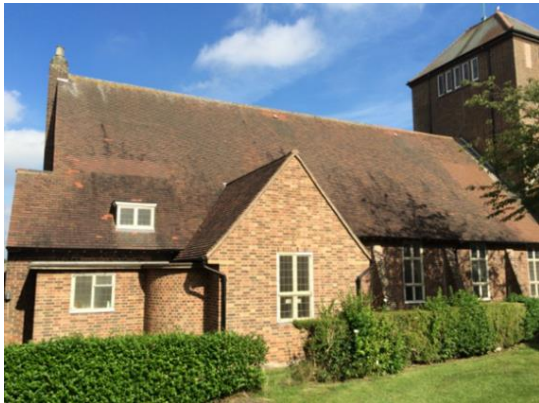
The old tiles being removed
